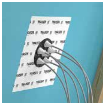
Timber frame construction. Panel construction.
