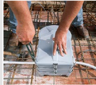
Also secure the housing to the reinforcement.
