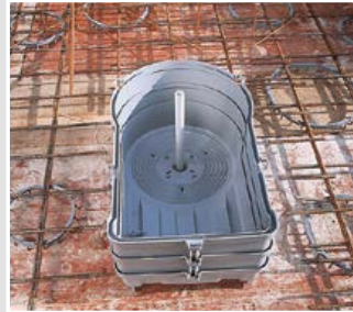
Attach the housing with 2 intermediate frames and a support conduit to the formwork.
