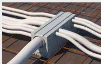
Numerous entries for conduits from Ø 20 mm to Ø 63 mm.
