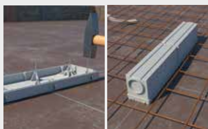
If required, several central transition casings can be lined up next to each other.
