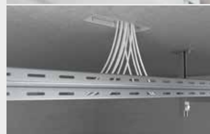
The central transition casing for the exit of several electric cables.
