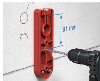
Drill the first centring hole through the guide hole in the drilling template at a distance of 91 mm.
