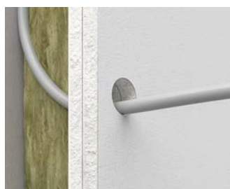
Cut an installation opening Ø 20 mm using a cutter (e.g. KAISER hardened metal cutter Art. No. 1088-06) or drill.
