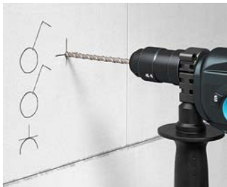
Drill the first hole Ø 6 mm at the intended position.
