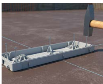
Fixing by means of steel nails.
