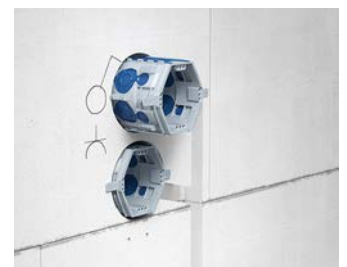
Insert the flush-mounted boxes.
