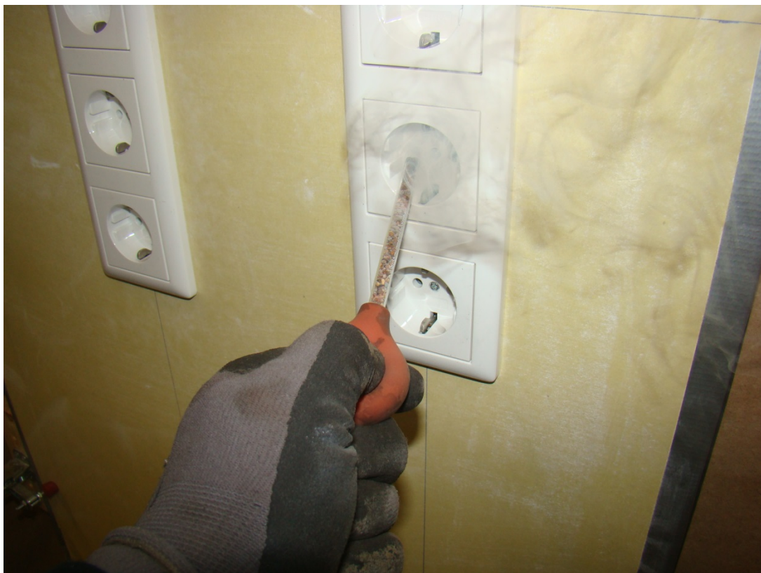
Picture B.4 S_{200} test, determination of leakages
