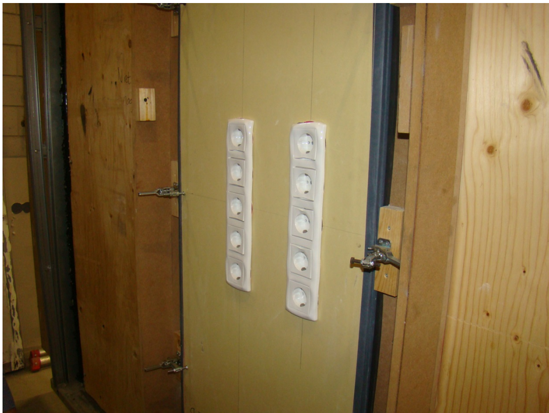
Picture B.5 S_{200} test, heated panel, deformation socket outlets
